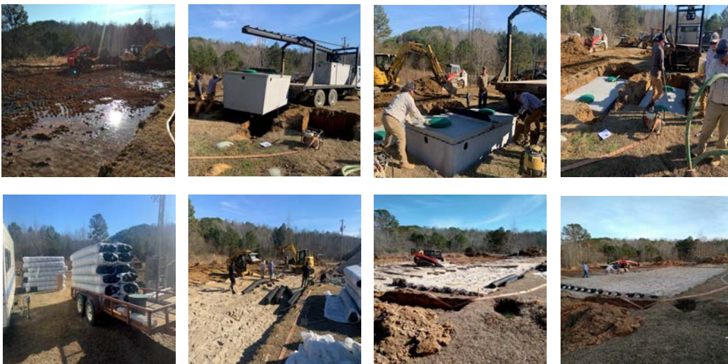
Infiltrator ATL Sand Bed Filter System being installed.
